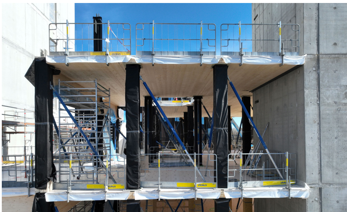
Wood and concrete. The wooden structure rises floor by floor. Photo: DTU
