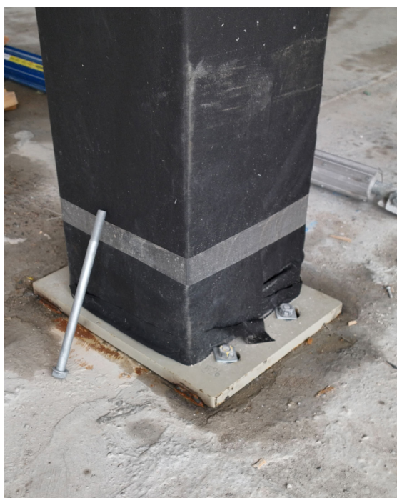
Precision work. The concrete deck acts as a foundation for the tree-house. On site, bolts are molded into the concrete and they must fit with the columns' pre-assembled fittings. Photo: DTU
