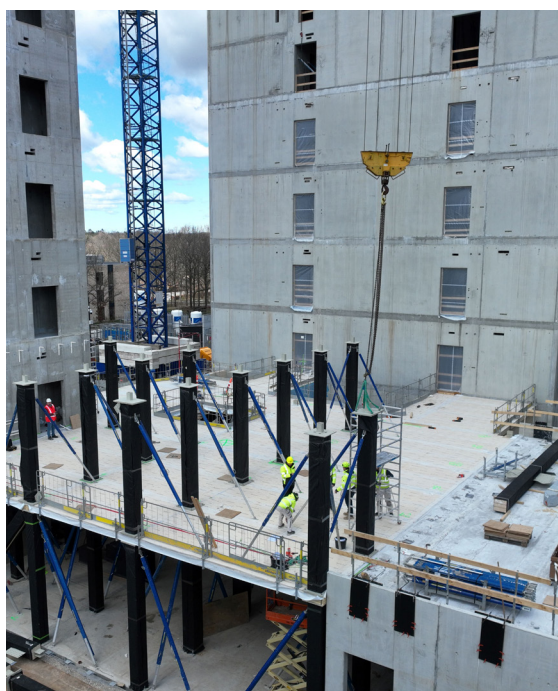
On site. CLT Denmark produces the wooden columns and installs the fittings at a factory. The CLT elements are delivered on trucks in the order they are to be installed on site (picture left). MT Højgaard hoists them off directly from the wagon in a special lifting device (picture right) developed to ensure the elements are lowered straight down and are easy to dismantle for a carpenter. Photo: DTU
